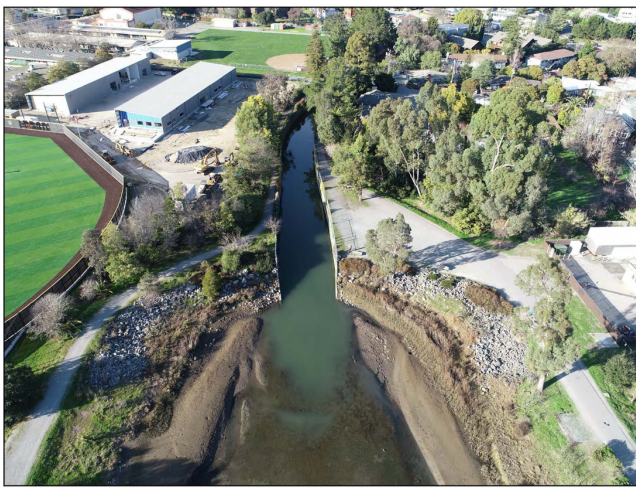
EXISTING CONDITIONS DATE OF FLIGHT: 5 FEB 2019 AT LOW TIDE (-0.3') (CONCRETE WALLS PREVENTS TIDE LEVEL FROM RISING BELOW 1.7' IN CONCRETE CHANNEL)
